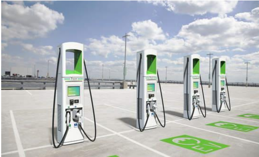
Figure 11: EV charging stations
