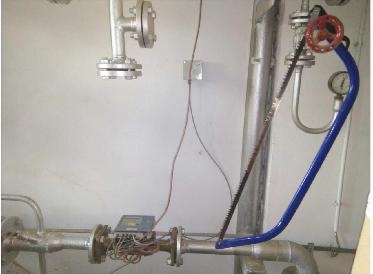
Device for heat energy reading
