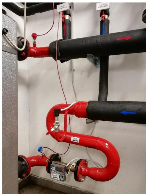
*Picture 6: Built-in heat meter for measuring the consumption of heat produced.*
