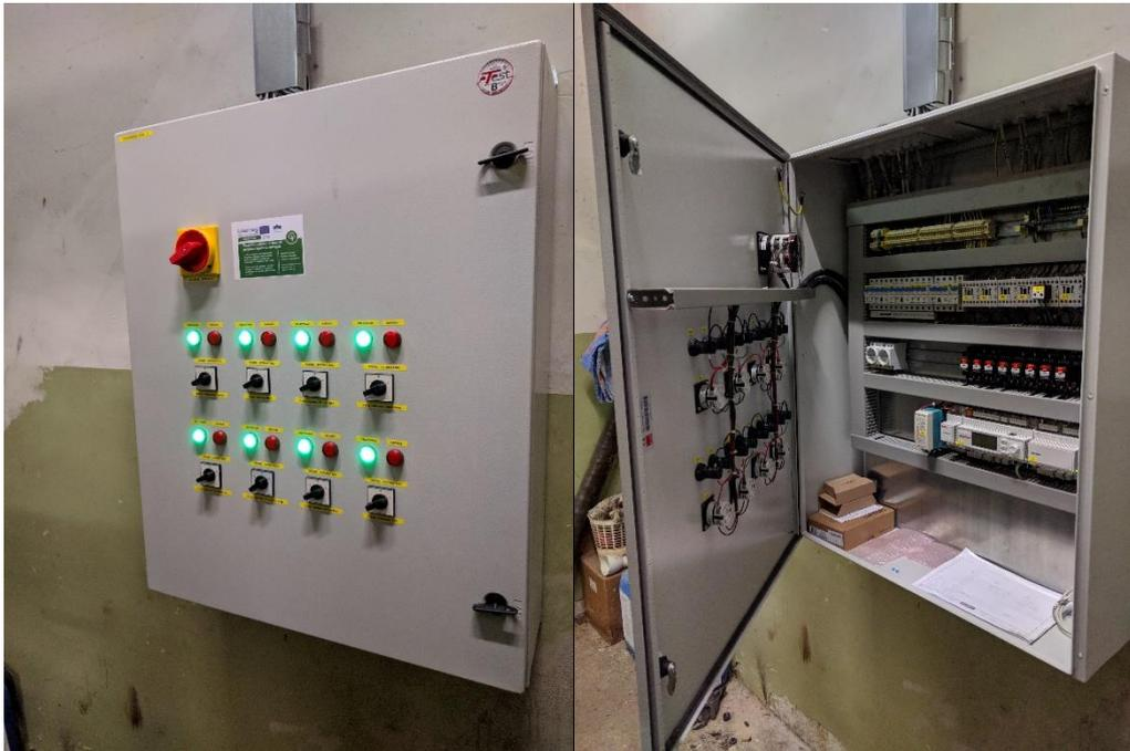
*Picture 23: Built-in main cabinet to control the operation of the entire boiler room.*
