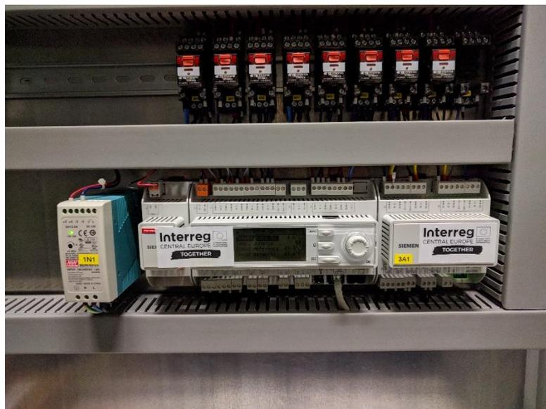
*Picture 24: Built-in smart controller for controlling the entire boiler room for the heat preparation for heating and sanitary water.*
