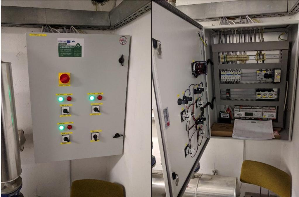
*Picture 30: Built-in main cabinet to control the operation of the entire boiler room.*
