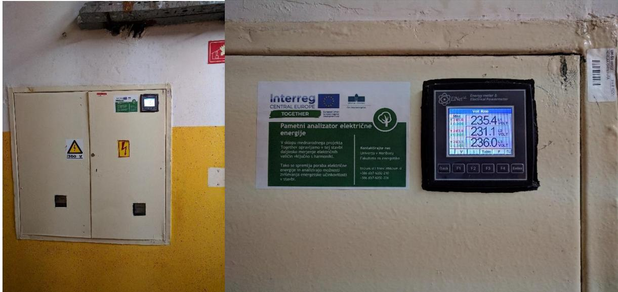
Picture 17: An updated electric cabinet on the ground floor with a smart power analyser.
