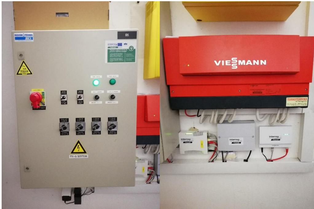
*Picture 7: An updated cabinet for controlling the operation of the entire boiler room (on the left) and an updated Viessman gas boiler with an expansion module (on the right).*
