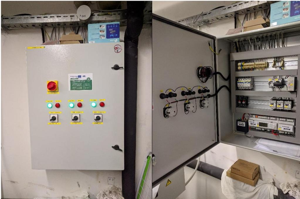
*Picture 15: Built-in main cabinet to control the operation of the entire boiler room.*
