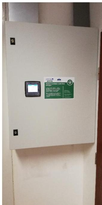
*Picture 8: An updated electric cabinet on the ground floor with a smart power analyzer.*
