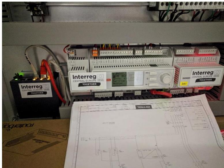
*Picture 31: Built-in smart controller for controlling the entire boiler room for the heat preparation for heating and sanitary water.*
