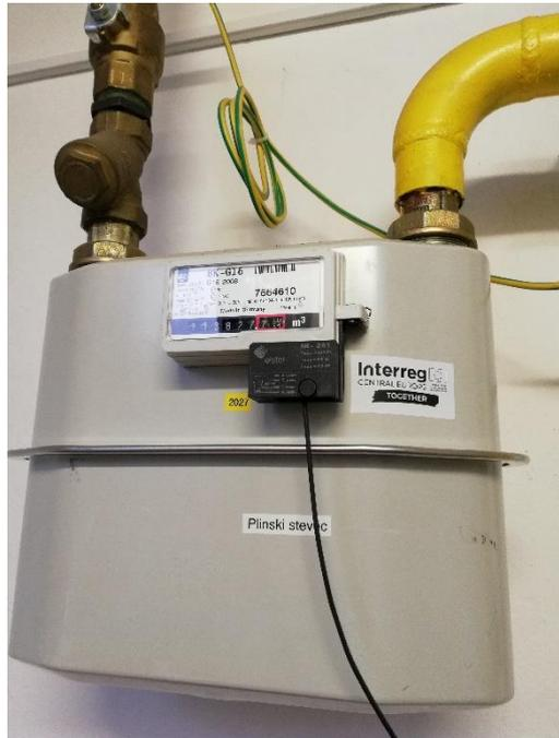
*Picture 5: Integrated incremental encoder for measuring energy consumption / natural gas consumption.*
