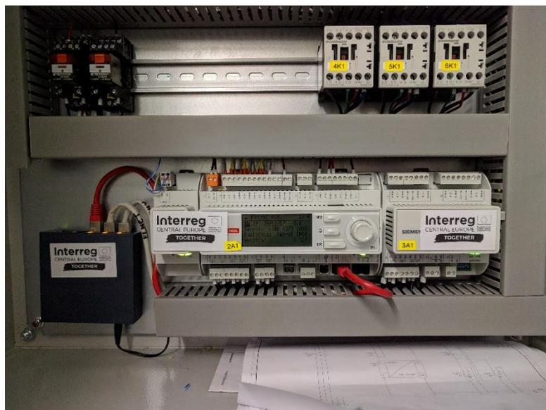
*Picture 16: Built-in smart controller for controlling the entire boiler room for the heat preparation for heating and sanitary water.*
