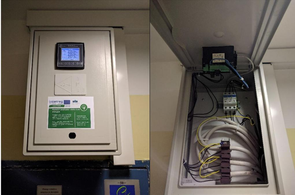
Picture 32: Integrated electric cabinet on the ground floor with a smart power analyser.
