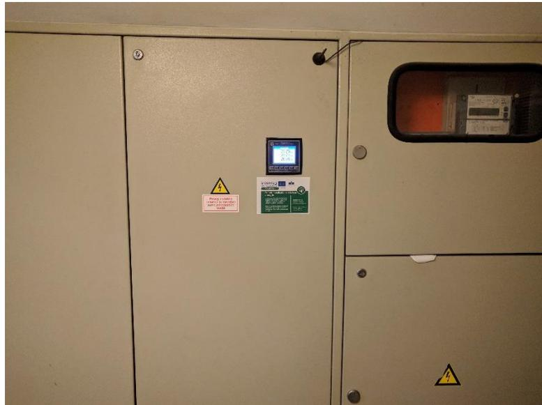
*Picture 25: An updated electric cabinet on the ground floor with a smart power analyser.*
