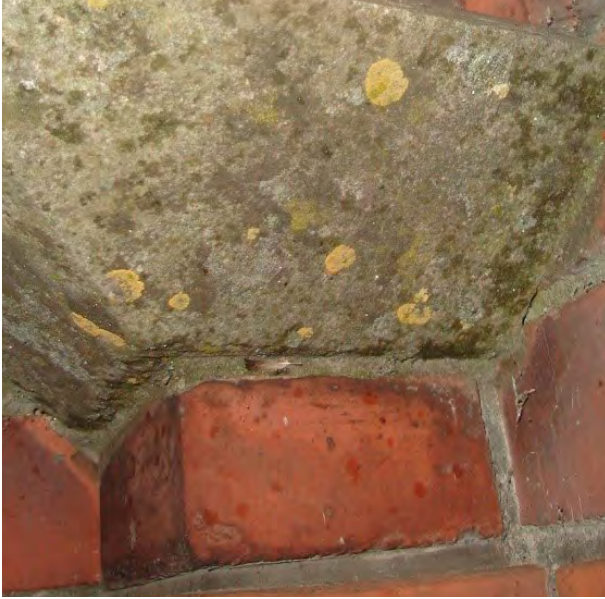
Photo 25. A fragment of a plastered ceiling overgrown with lichens.
