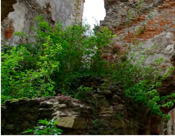
Photo 35. A fragment of the vault intensely overgrown with shrubs.
