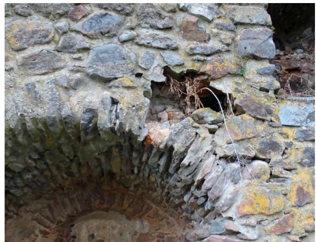
Photo 30. Damage to the face of the wall associated with the growth of the root system of low vegetation.
