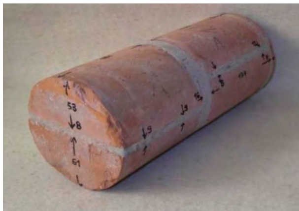
Photo 41. A core through the thickness of the wall. 18
