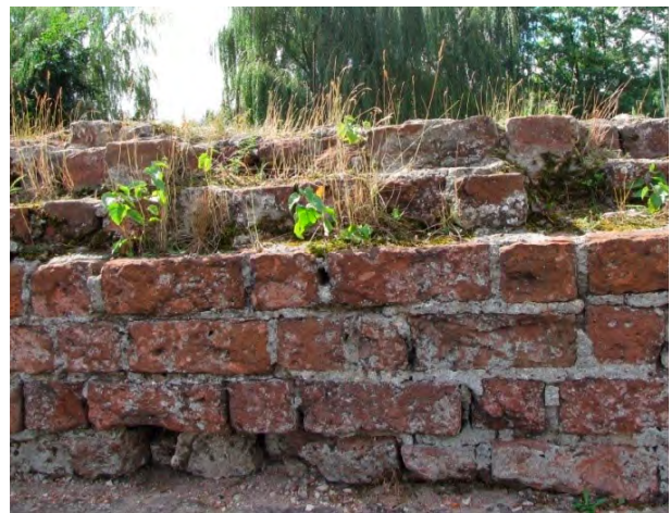
Photo 32. The expansion of low plants and mosses on the crown of a ceramic brick wall. In the foreground young shrubs are visible.
