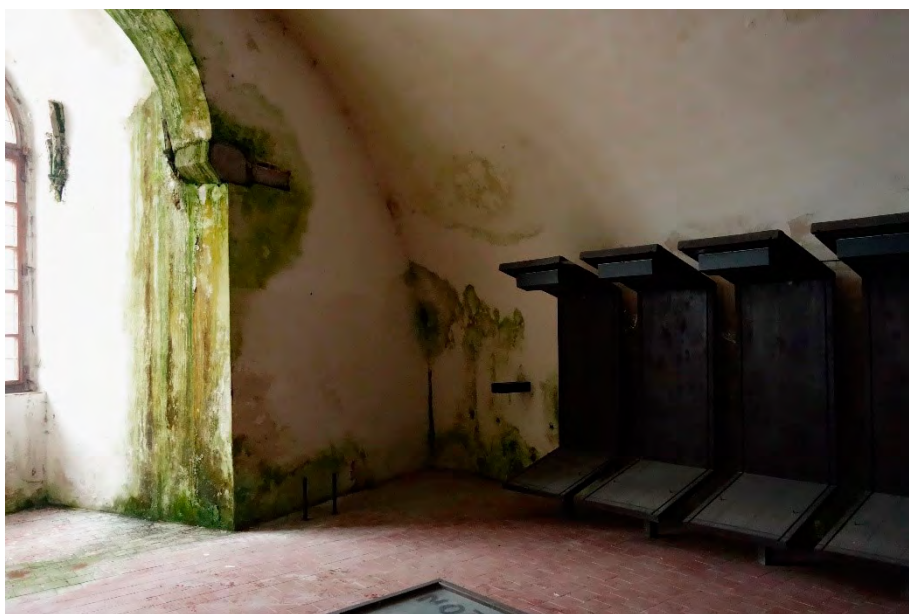
High humidity in the interior of the Great Tower (photo Lucie Bláhová 2017)
