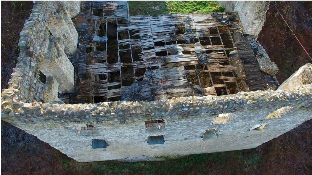
Photo 3. A photo of a wall crown made with the help of a drone.
