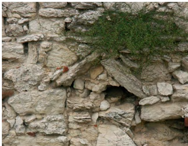
Photo 29. Photograph of a heavily sunlit southern façade. The development of vegetation in the wall crevices.
