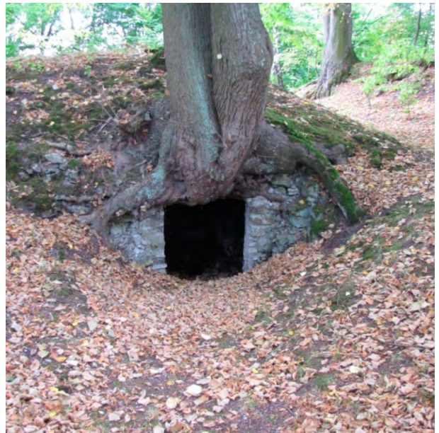
Photo 40. A huge tree and its root system, which has overgrown a stone vault.
