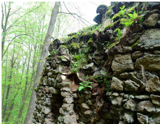
Photo 31. The crown and the face of a curtain wall overgrown with annual and perennial vegetation.
