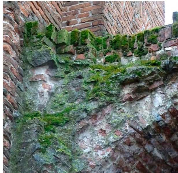
Photo 28. Moss and algae, which overgrow the crown and the face of the wall.
