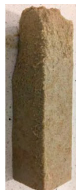
Photo 70. Frost resistance test. A sandstone sample after 30 freezing cycles. 3rd degree damage
