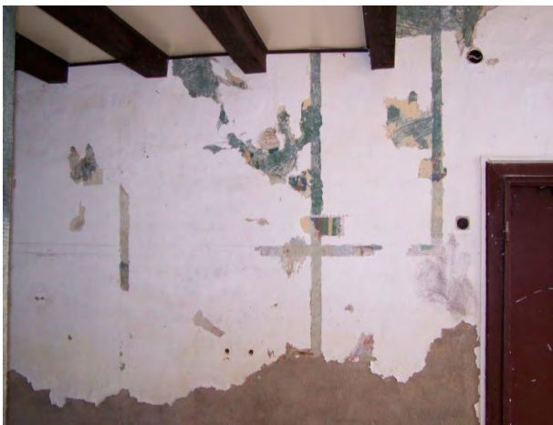
Photo 21. Strip outcrop with probes revealing bottom layers of painting.
