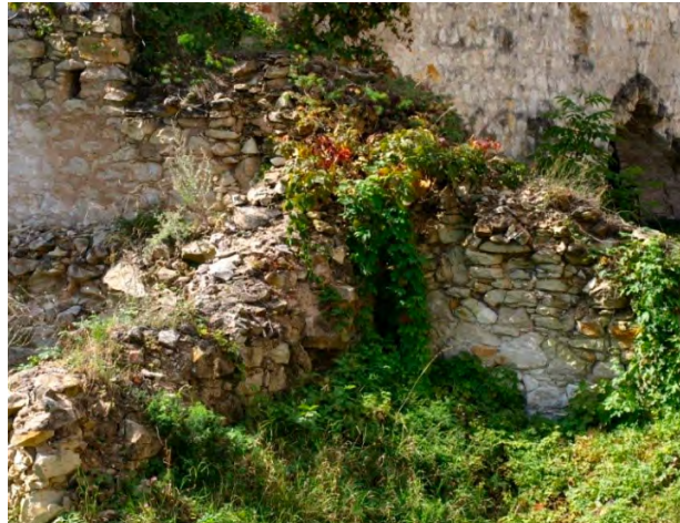
Photo 34. A wall relic covered with vegetation. A large amount of greenery causes the illegibility of the ruin.
