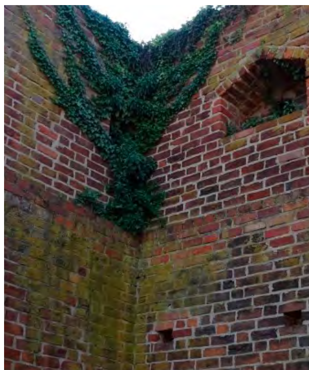
Photo 24. The development of algae and lichen in the corner of the wall directly under the ivy, which grows on the wall and the crown.
