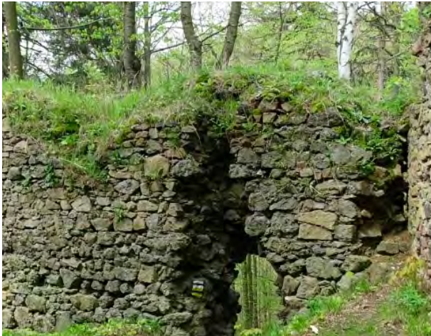
Photo 33. The low crown of the wall completely overgrown with greenery. The tight layer of humus and greenery prevents evaporation of the moisture retained in the wall.
