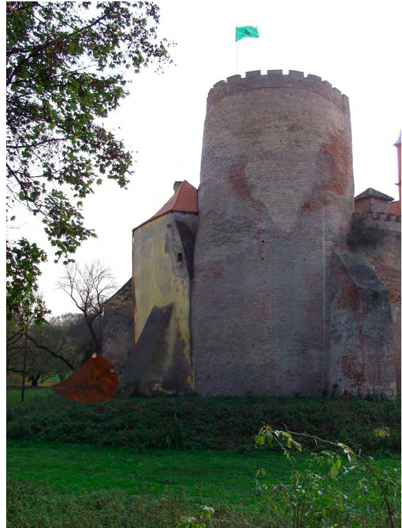
Picture 10. The present state of the tower: the “stains” on top of the walls indicate the restored parts of the tower as well as areas with increased amounts of moisture in the walls
