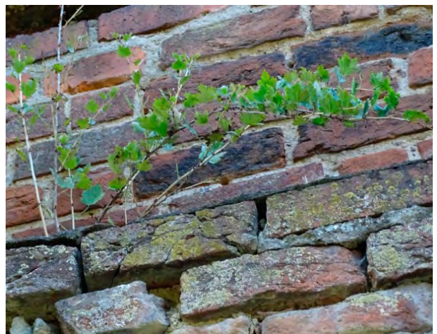
Photo 38. A shrub with a root system growing into a ceramic brick wall
