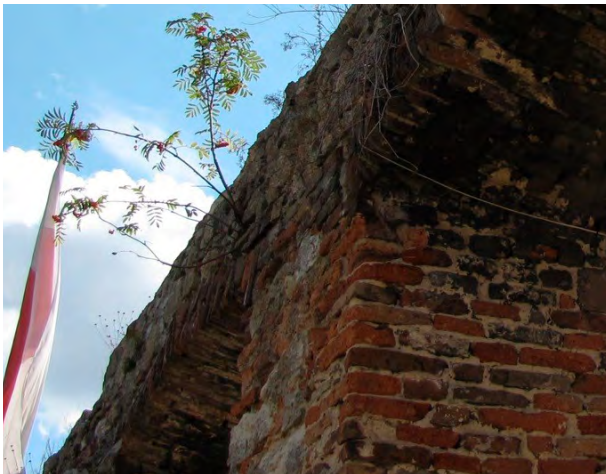
Photo 37. The rowan rooted in the gap between the wall of the crown and the lintel.
