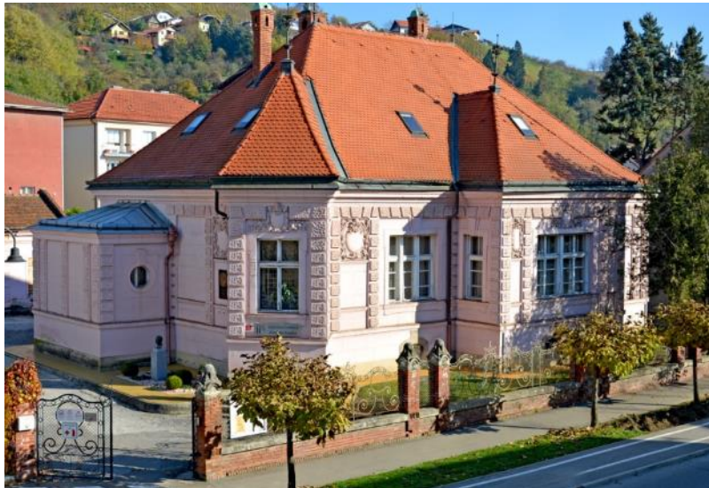
Figure 7: Pilot building in Lendava
