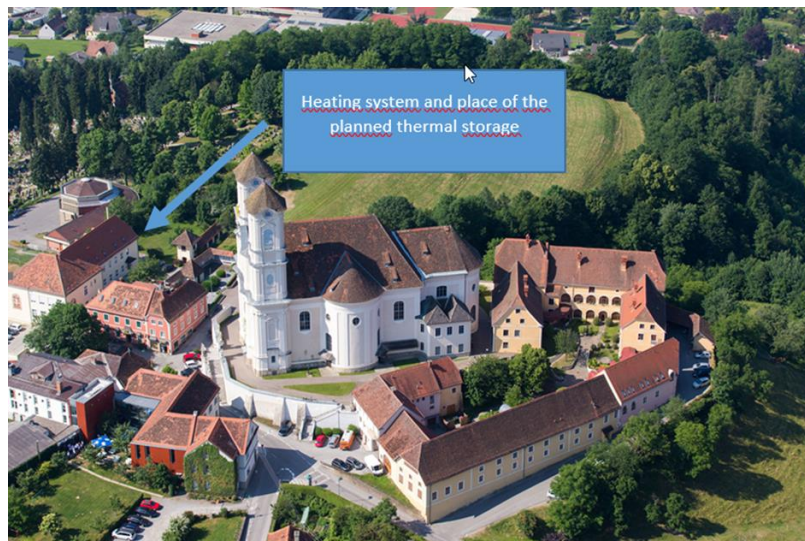
Figure 3: Location of the heating station where the storage will be installed
