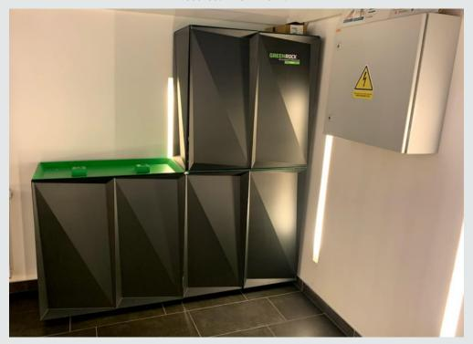
Figure 4: The storage (battery system) is placed in the premises of the Bračak Manor, in the basement next to the stairs.
