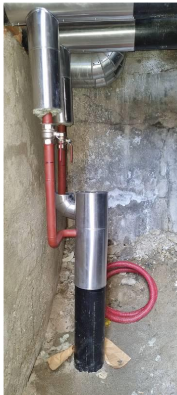
Figure 14: Construction work - connection of the new pipeline to the primary network
