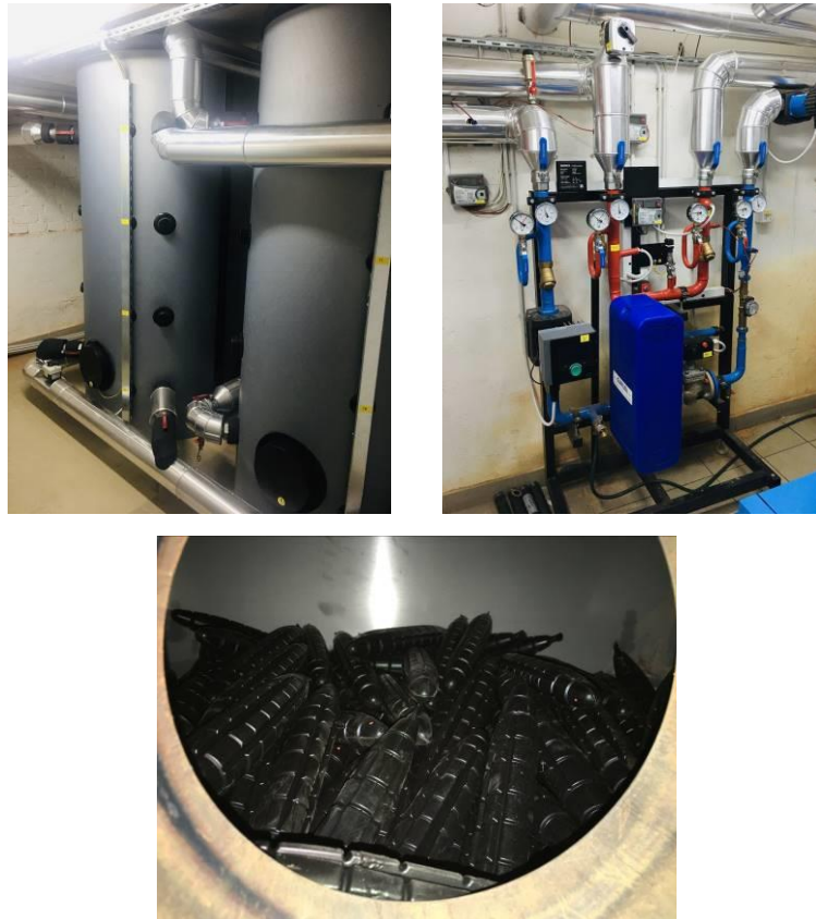
Figure 4: Installation of the storage tank with PCM material and all electrical and mechanical components for energy transmission and measurement
