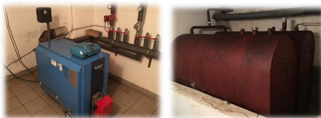
Figure 7: Existing inefficient old heating oil boiler
