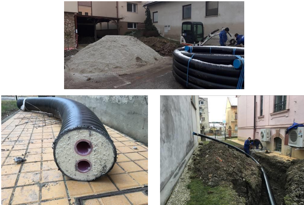
Figure 3: Construction work - pipelaying and connection of the building to the geothermal network
