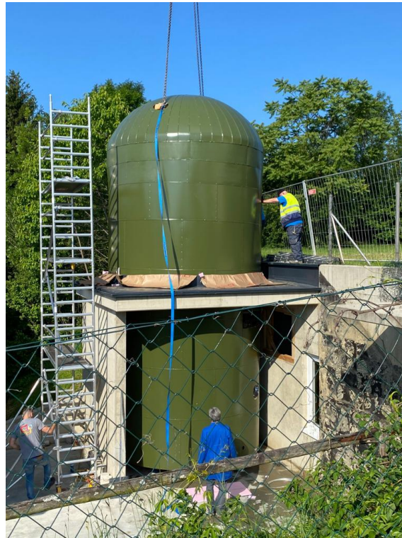
Figure 1. Last work during the storage installation
