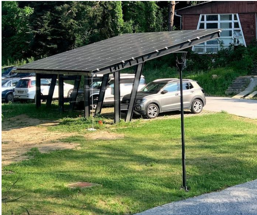
Figure 3: Installed photovoltaic modules
