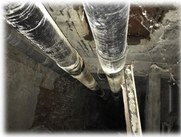
Figure 14: Existing district heating pipeline under the pavement at Kranjčeva street - new connection location
