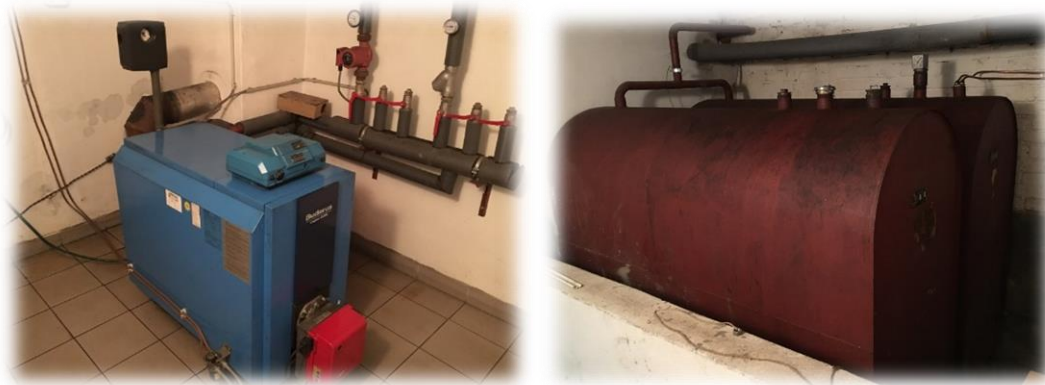
Figure 7: Existing inefficient old heating oil boiler
