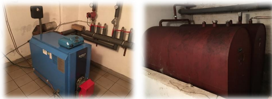
Figure 6: Existing inefficient old heating oil boiler and the heating oil storage tank
