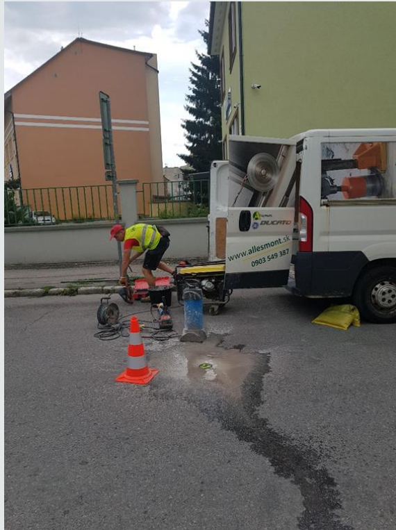
Figure 1: The road surface installation of smart sensors of traffic flow
