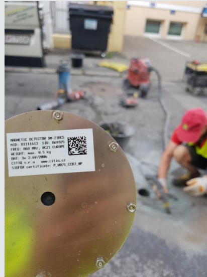
Figure 1: The road surface installation of smart sensors of traffic flow
