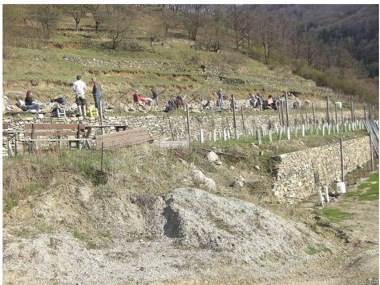
Figure 2 Dry-stone walls in the Wachau. ©Rainer Vogler
