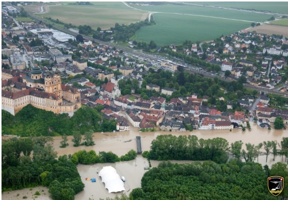
Figure 7 Flooded old city of Melk, on the left the monastery. © ÖBH Kermer.
