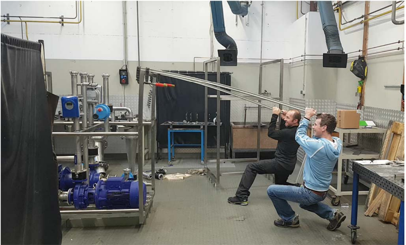
Figure 1: Building the pilot plant
