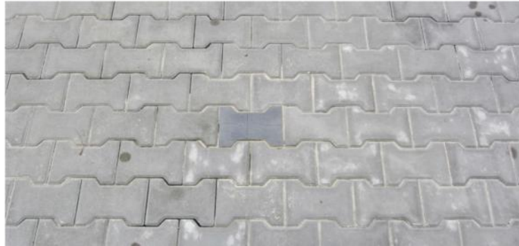
Figure 12: Magnetometer illustration; integration into a pavement cobble (Source: CDV, v. v. i and CITIQ, s.r.o.)
