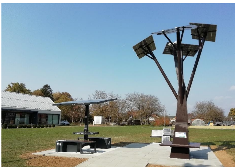
Image 11 Finalised Solar E-Tree installation
