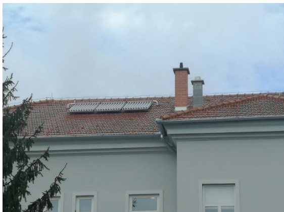
Image 20 Solar collectors for hot water and heating support
