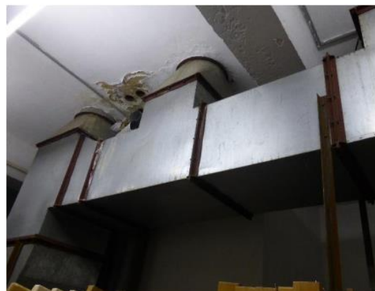
Image 4 Old ventilation system
