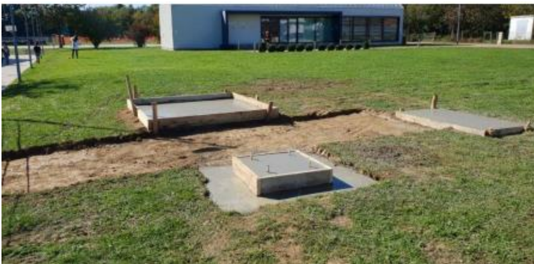
Image 10 Preparation of the foundation
