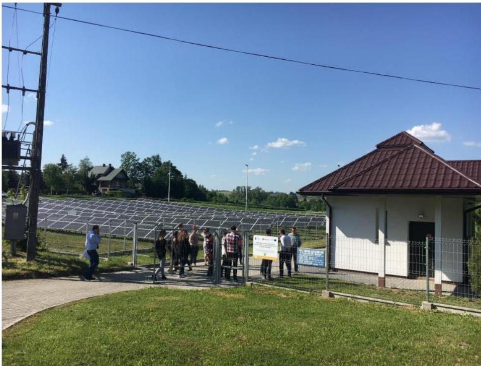
Image 5 PV installation near water pumping system
