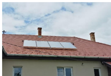
Image 12 Solar system for hot water
