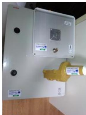
Image 8 New water meter and equipment
