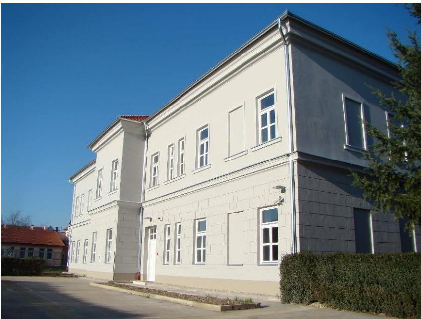
Image 16 Building where Croatian pilot installations are located
