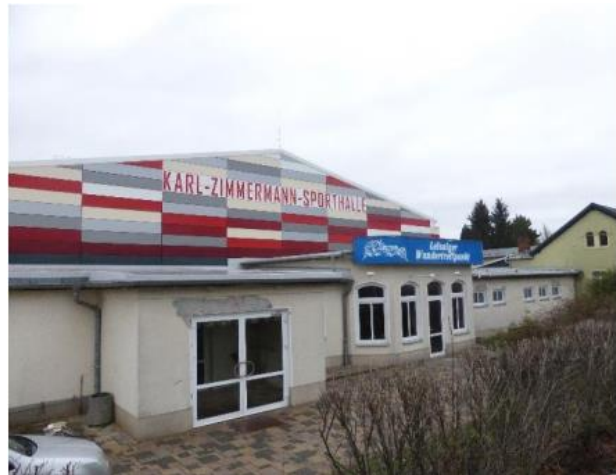
Image 2 Street view of the sports hall
