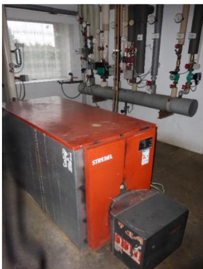
Image 3 Old heating system
