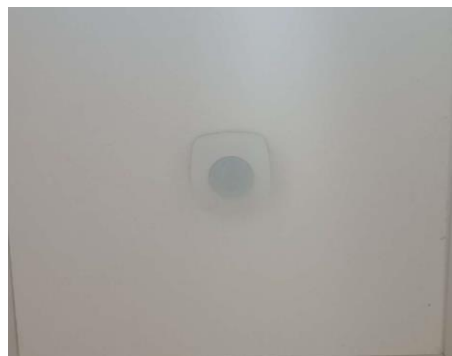
Image 17 Installed movement sensors
