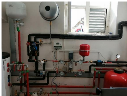
Image 19 Additional technical equipment for solar water heating
