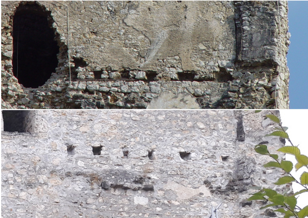
Photo 9 Šalek castle – same detail of the wall before & after the wall reinforcement (photo Rok Poles)
