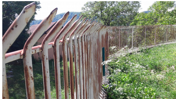
Photo 6 The fencing is designed in an aggressive way
