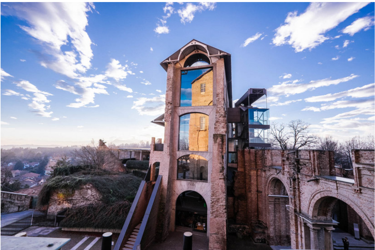
Picture 9: compatible reuse of the Castle of Rivoli (Italy), transformed into a Museum of Contemporary Art by Andrea Bruno. The general criterion of intervention was to bring the Castle back to the "unfinished" situation, typical of the unfinished building site of Juvarra at the time of its interruption, without completions or remaking, so that everything belonging to the past time was kept in its authenticity, both historical and artistic.
