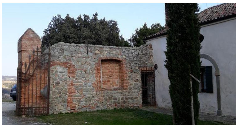
Picture 29: Detail of the northern wall of the monumental complex, which has been identified as the northern wall of the ancient medieval church of the monastery. In the wall, a niche and a walled door are visible.
