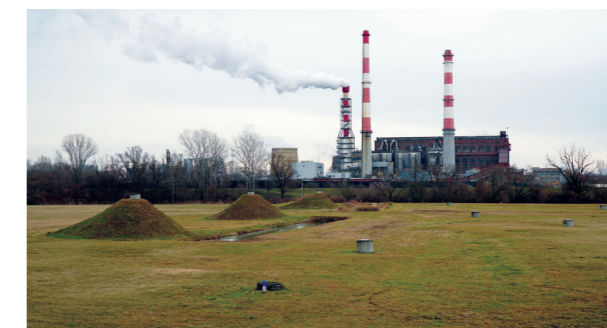
POLAND Tarnów Waterworks
