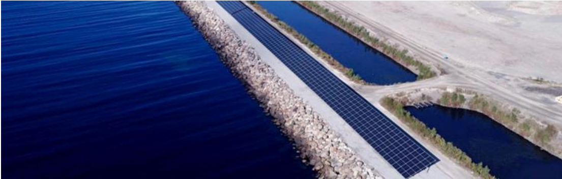
Solar panels at the new quay © Port of Trelleborg
