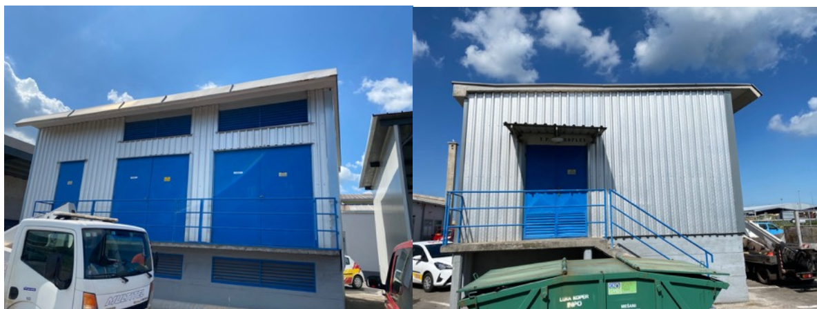
Figure: Existing transformer station
