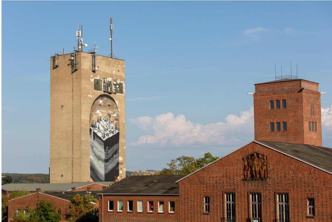
Picture 2: Art installation on the shaft tower (Picture Thomas Dietze)
