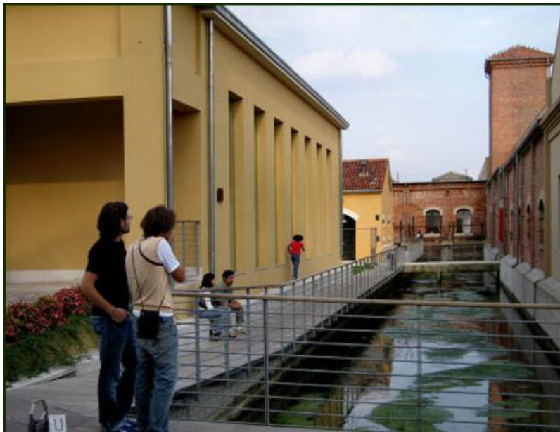
Picture 3: Site of the social innovation centre (Picture Camera die Commercio Padova)
