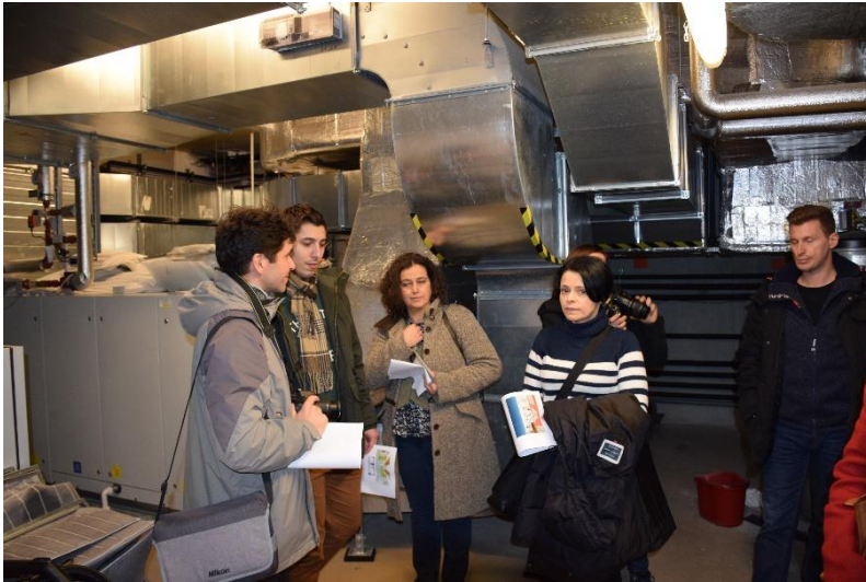
Figure 7. MEP room (source: InAirQ team)
