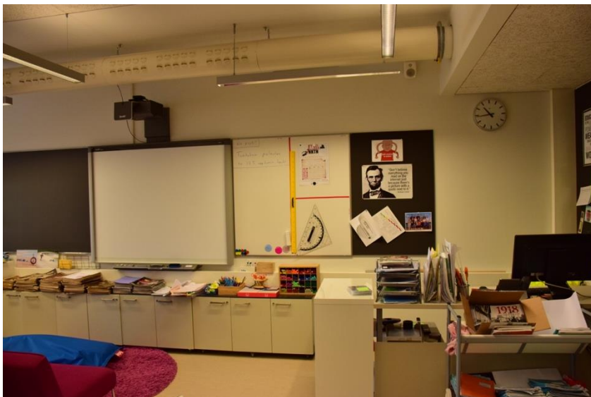
Figure 24. Classroom: mechanical ventilation (source: InAirQ team)
