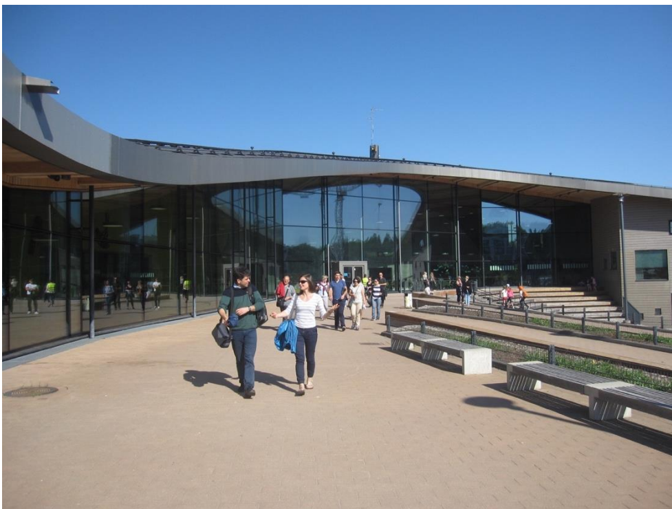
Figure 28. Glass façade (source: InAirQ team)
