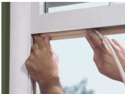
Figure 15: Weatherstripping window (www.berwickelectric.com)
