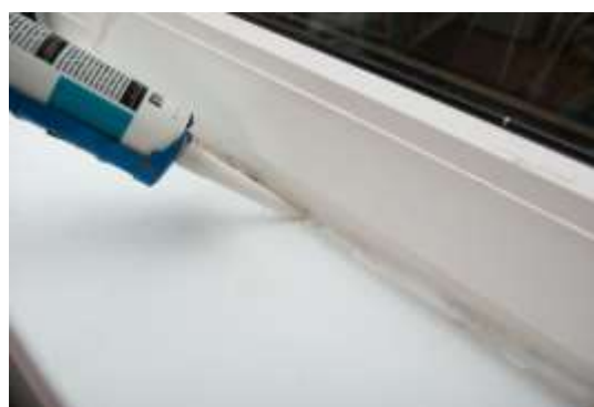
Figure 14: Caulking window ( www.delfera.com )
