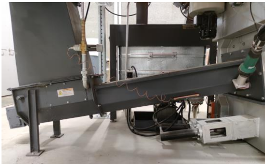
Figure 6.35 Feeding with screw conveyor (source: Schmid energy solutions).
