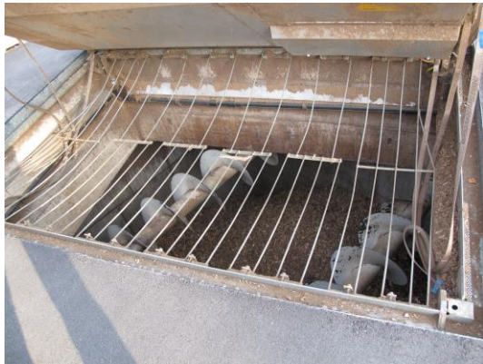
Figure 6.11 Filling screws (source: Holzenergie Schweiz).
