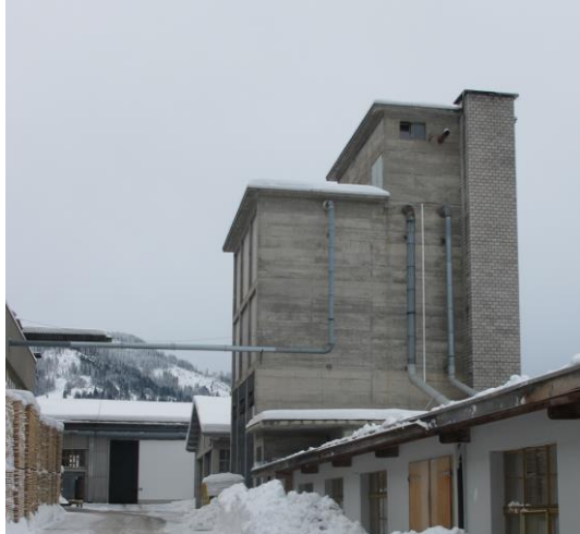
Figure 6.4 Chips silo (Source: Wooden Energy Switzerland).
