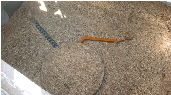
Figure 6.27 Discharge system with articulated arm for quality wood chips and pellets (source: Holz-energie Schweiz).
