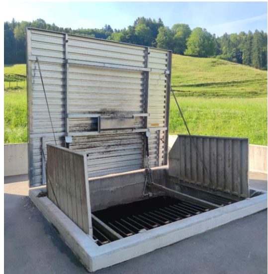
Figure 6.8 Silo lid not accessible when open (source: Schmid energy solutions).
