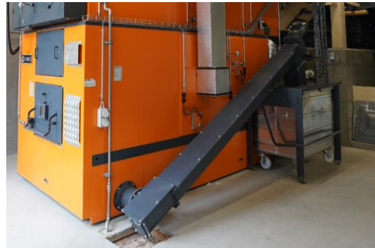
Figure 6.39 Fire ash screw (source: Schmid AG energy solutions).
