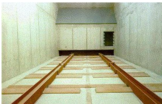
Figure 6.21 Silo discharge by push floor (source: Schmid energy solutions).
