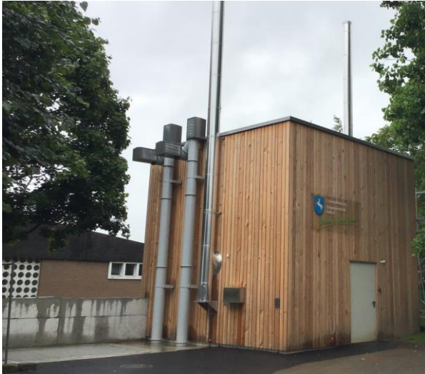
Figure 13.32 Central heating plant as prefabricated element with integrated or additional fuel storage tanks (source: Holzenergie Schweiz).
