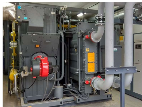
1,25 MW direct fired HP
