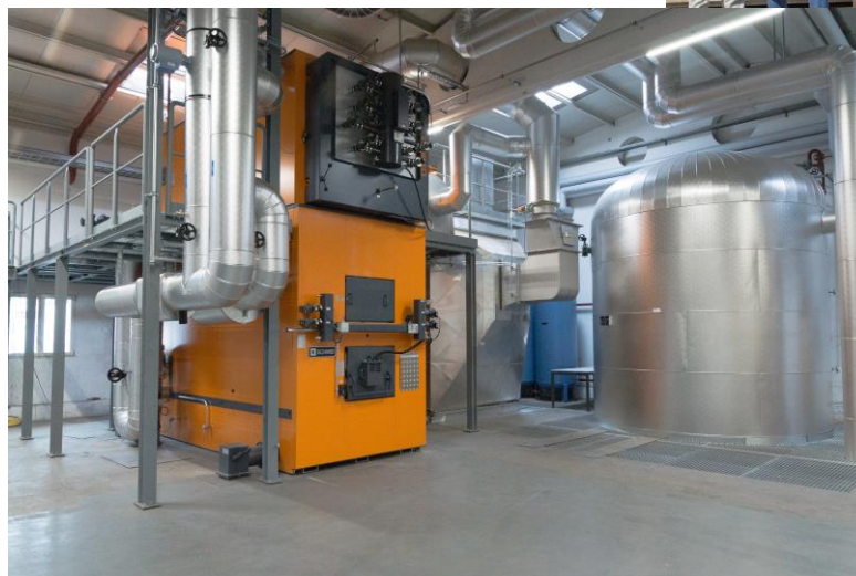
Schmid energy solutions
