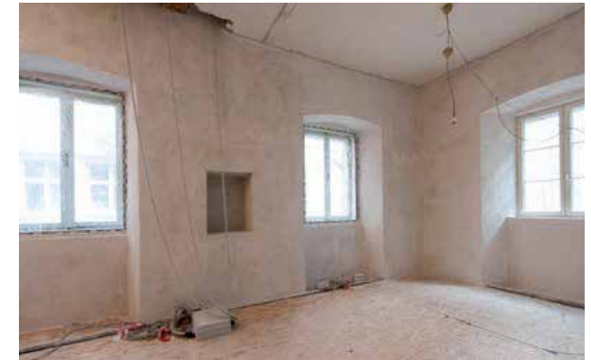
Isolation from the inside of an historic wall.
