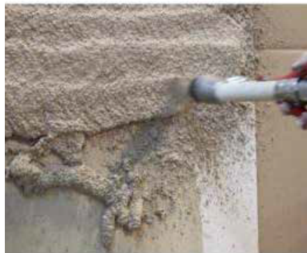
Application of thermal insulating plasters that provide insulating properties.
