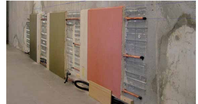
Plant system temperierung in phase of installation.
