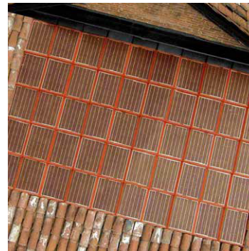
Integration of photovoltaic panels into the roof of historic buildings
