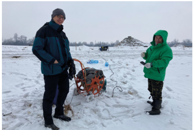
Cleansing pumping of a piezometer
