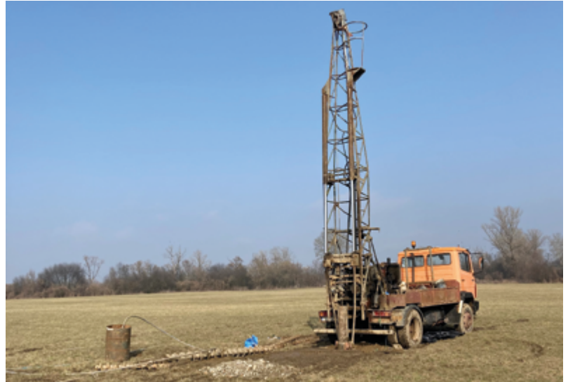
Drilling of piezometers to collect water and soil samples
