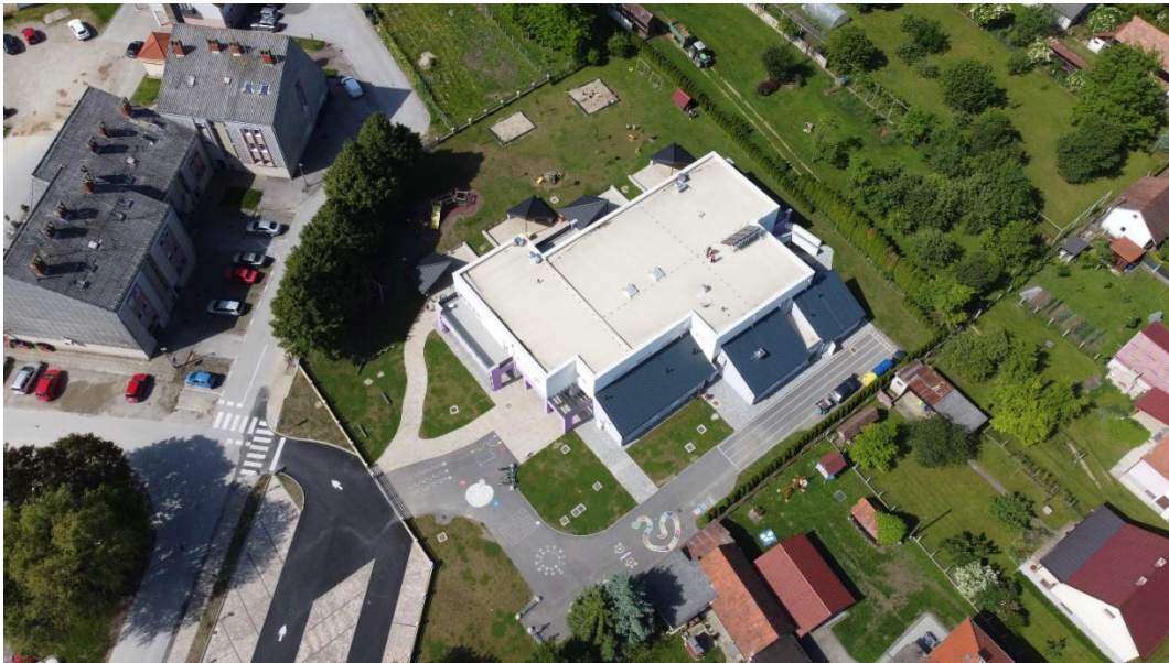
Image 9 Roof area of the Kindergarten "Fijolica" in Prelog
