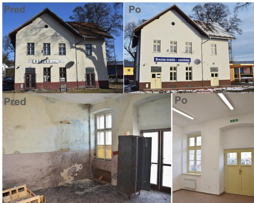
Fig 11 – Building before and after renovation works
