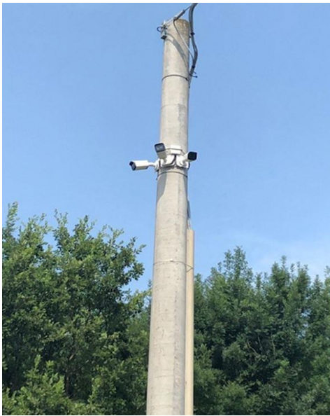
Fig. 11a,b - Three video-cameras system setting, placed on an existing pole (on the left), and the industrial PC embedding the software for images acquisition and processing with Artificial Intelligence features (on the top right of the right photo).
