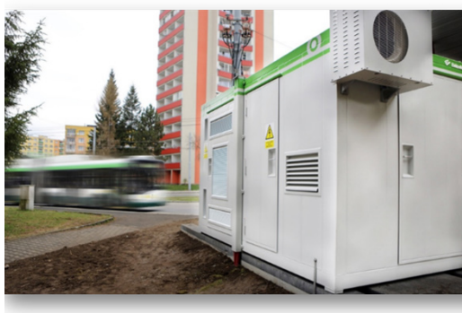
Figure 10 PMDP tested a buffer storage station with an IMC Trolleybus to replace Diesel buses. Source: PMDP.
