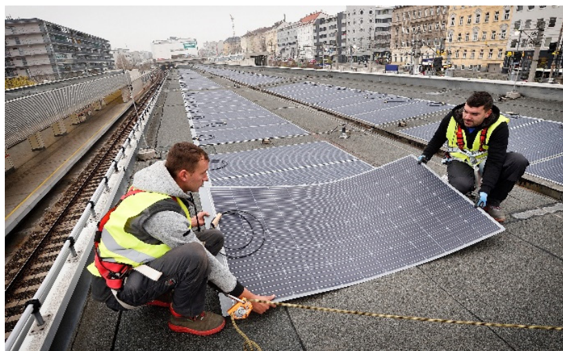
Figure 6: PV foil installation in Vienna. Source: WL.
