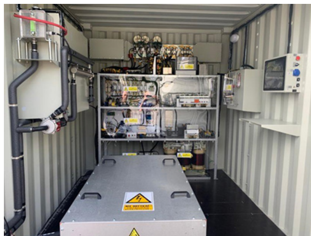
Figure 5: Battery-based electric energy storage; usage of a second-life traction battery from a trolleybus. Source: PKT.
