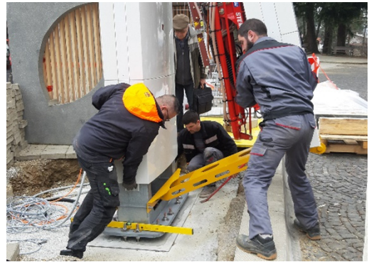
Figure 15 Installation of fast charger in Maribor. Source: City of Maribor.
