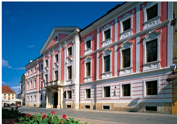
Photo 2. View of the main facade of Varaždin County Palace (present condition)
