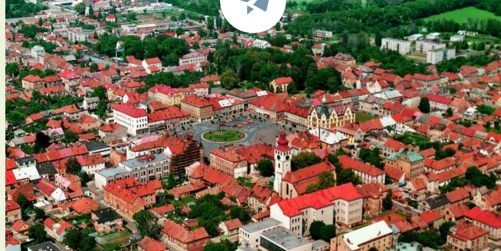
Figure No. 20 - The aerial photo of the town centre
