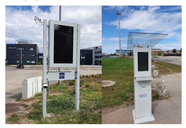
1. Figure Installed devices for the smart access and traffic management system
