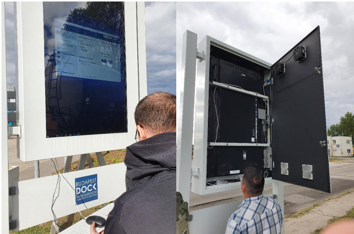
4. Figure: Installation and implementation on-site of FBL
