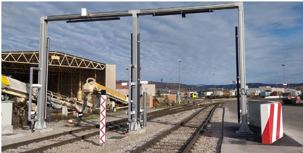
Figure 3: installed OCR system in the port of Koper (Source: Luka Koper's archive)
