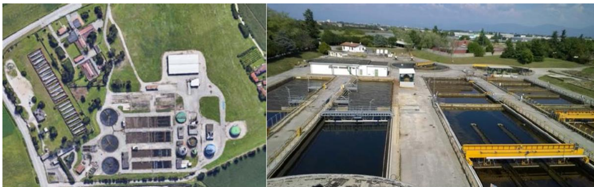
Figure 4: CAFC S.p.A. (waste-water treatment plant)
