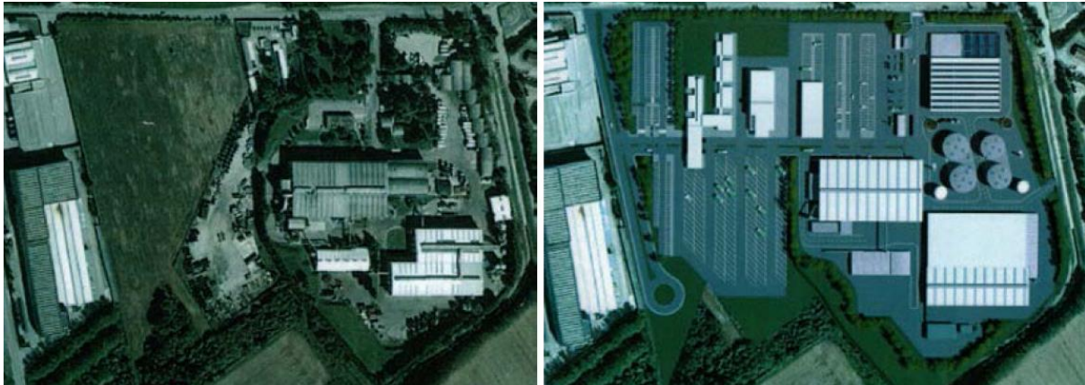
Figure 5: NET S.p.A. (organic-waste treatment plant), existing (left) and rendering after foreseen enlargement (right)
