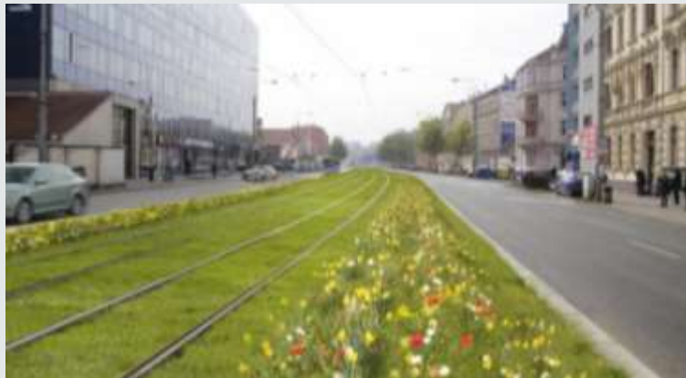
Figure 19: Visualization of reconstruction of tram lines Nové sady in Brno, where the “green belt” - meadow lawn with flowers - will be built for less noise and dust. Source: www.dpmb.cz
