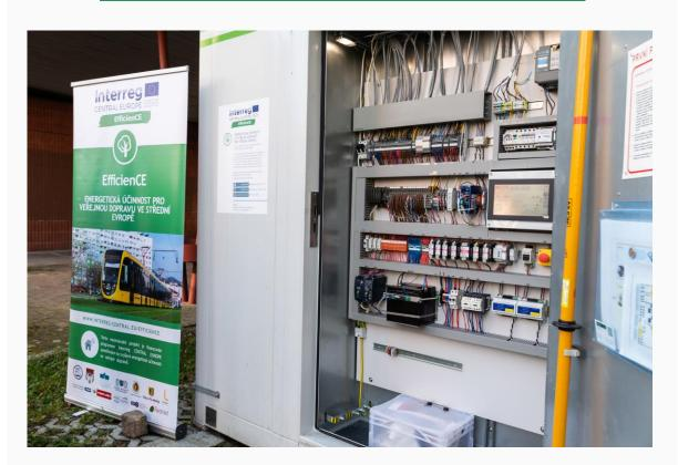
The Pilsen City Transport Company (PMDP) has launched a series of tests of a battery buffer storage station at the final station of trolleybus line 16. This interesting technology will fit the dimensions of a small shipping container. The main function of the station is to strengthen places with insufficient power supply. >> Read more HERE.
