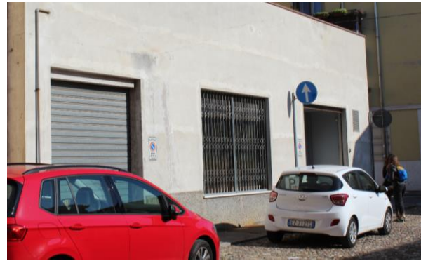
Bicycle warehouse via Gradaro
