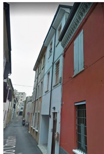
Figura 13 rebuilt house on gothic plot
