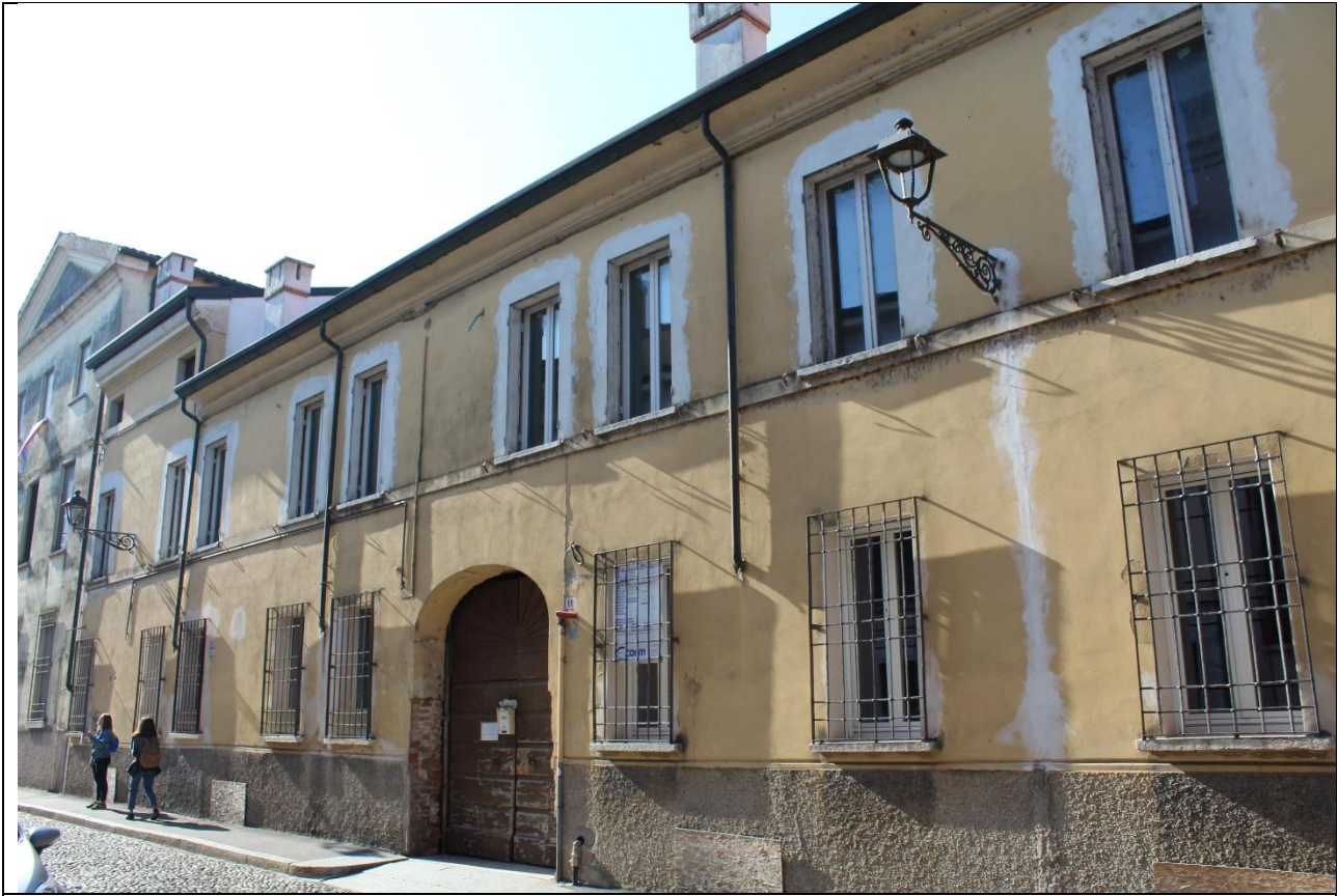
B71 – Building already detected as construction site in the year 2012
