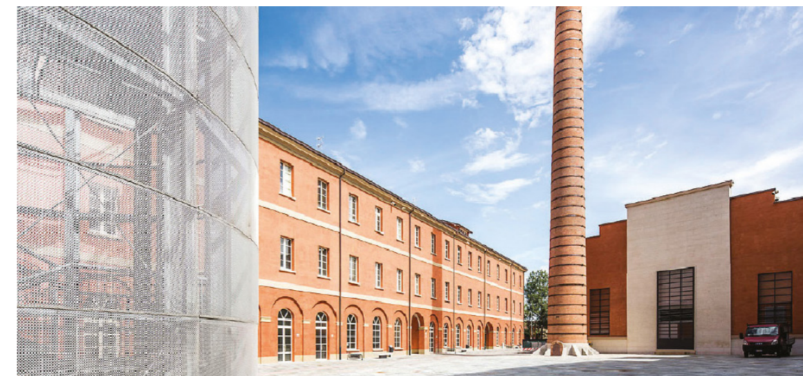
Exemple of a recovery building factory. Manifattura Tabacchi, Modena.
